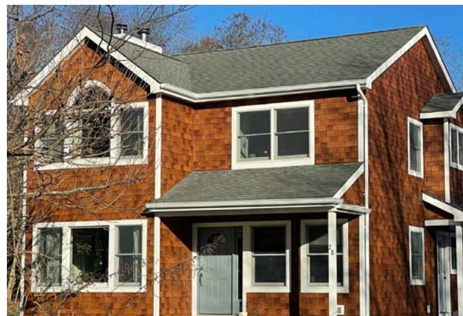
AFTER With Beach House Shake Pacifica Installed
